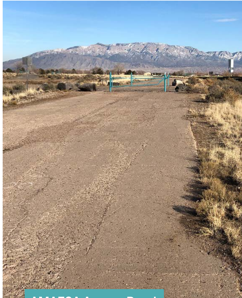
AMAFCA Access Road
